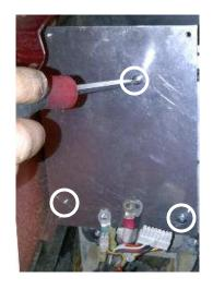
**2.** Using the original controllers mounting bolts and holes mount the conversion plate to the vehicle heatsink.
